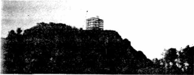
Framing the MMT high atop Hopkins.
